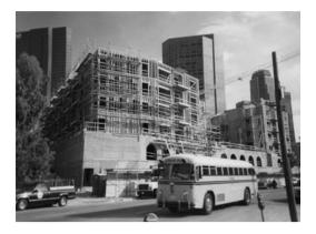
Figure 2. Apartment complex utilizing FRTW studs.
