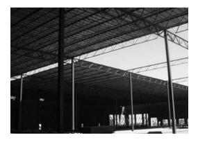
Figure 1. FRTW panelized roof system.
