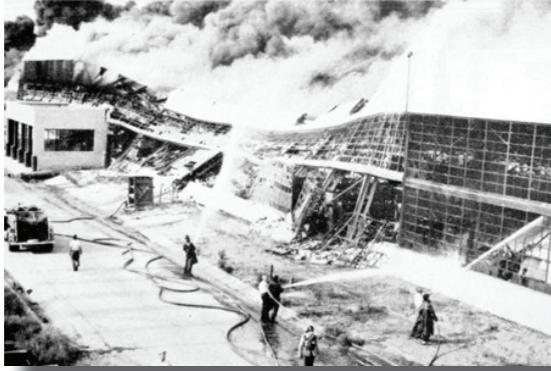
At one time, roof assemblies were assumed to be fire safe if the deck and its supports were of metal, particularly when the fire hazard of the building's contents were considered low to moderate. This type of roof construction was classed as "non-combustible" even though the vapor barrier, adhesive and roofing used were combustible.
