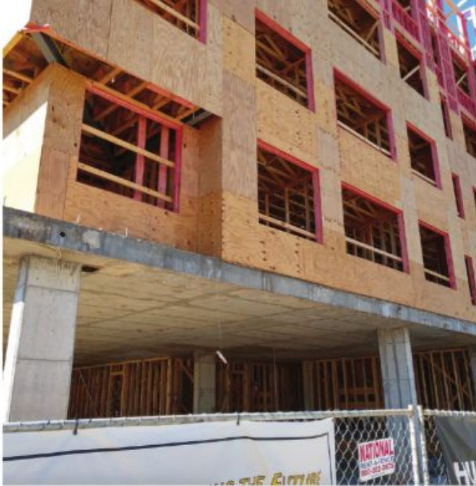
Type III with Type I podium: Interior FRTW used both above and below the podium in Charleston, South Carolina.
