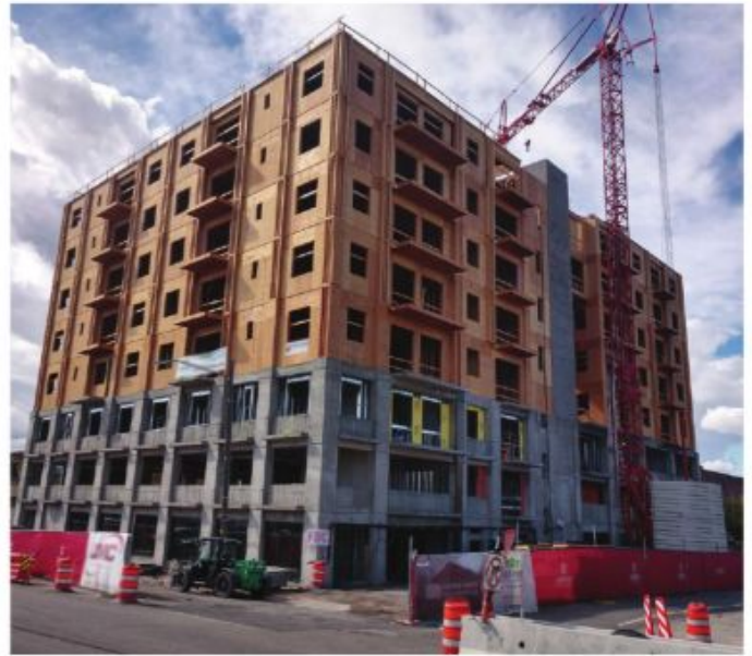
Type III with Type I podium: five-story interior FRTW used above three-story podium in Salt Lake City, UT.
