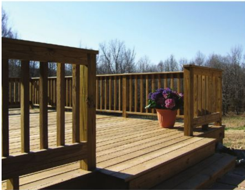
Exterior FRTW being used in the wildland urban interface (WUI) for decking.
