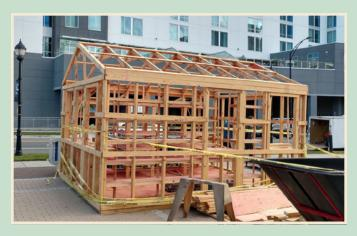
PyroGuard  $^{\rm TM}$  lumber and plywood are used for the construction of outdoor/mall kiosks. Charlotte, NC.
