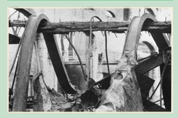
In 1953, a fire in a casein glue factory demonstrated the superior fire-endurance of untreated wood over steel.
