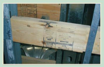
PyroGuard $^{\text{TM}}$  is frequently used as blocking in the walls of Type I and II construction. Cleveland, OH.
