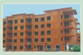
Type III: UL Design No. V314 used PyroGuard™ for the 2-hour bearing exterior walls in Draper, UT.
