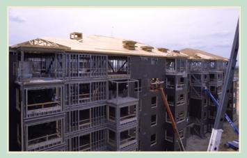
Type II: PyroGuard  $^{\text{II}}$  pitched roof system used as a nail base for 3D architectural shingles in Tulsa, OK.
