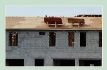
PyroGuard™ plywood used four feet on each side of a wall to eliminate parapets. St. Petersburg, FL.
