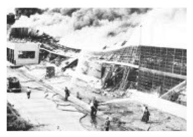
At one time, roof assemblies were assumed to be fire safe if the deck and it supports were of metal, particuarly when the fire hazard of the building's contents were considered low to moderate. The type of roof construction was classeed as "noncombusitble" even though the vapor barrier, adhesive and roofing used were combustible.
