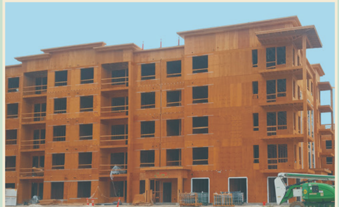
Type III: UL Design No. V314 used PyroGuard™ for the 2-hour bearing exterior walls in Draper, UT.
