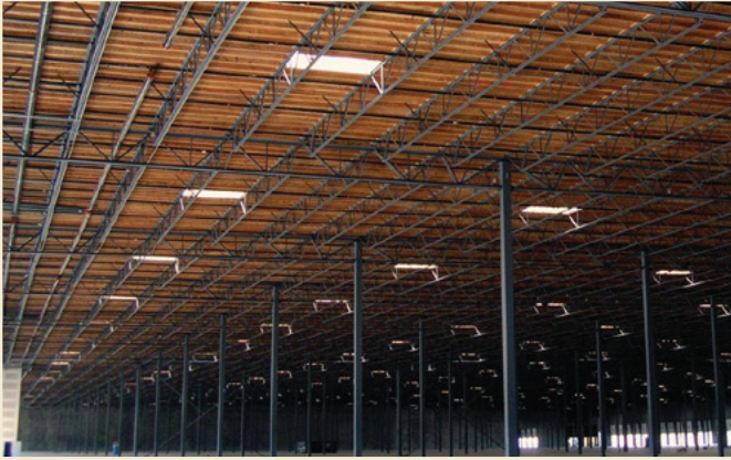
Type I: 1.2 million SF panelized roof system used PyroGuard™ lumber and plywood. Phoenix, AZ.
