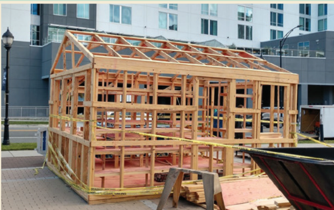
PyroGuard™ lumber and plywood are used for the construction of outdoor/mall kiosks. Charlotte, NC.
