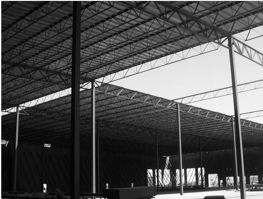
Modern 1.2 million square foot warehouse that features a hybrid panelized roof system utilizing fire-retardant-treated lumber and plywood.
